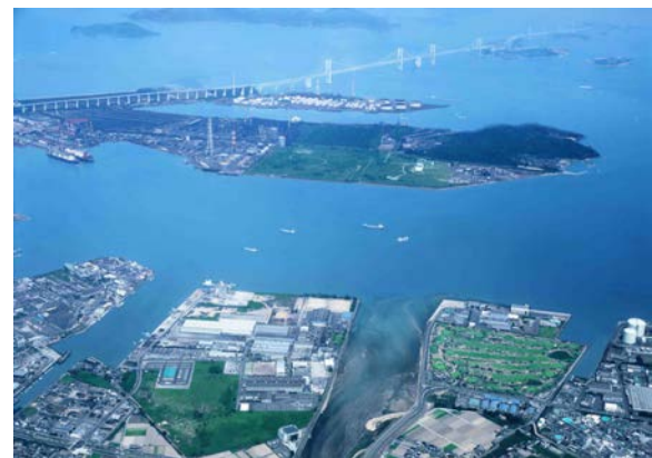
Sakaide Plant near Great Seto Bridge (Kagawa Pref.)
